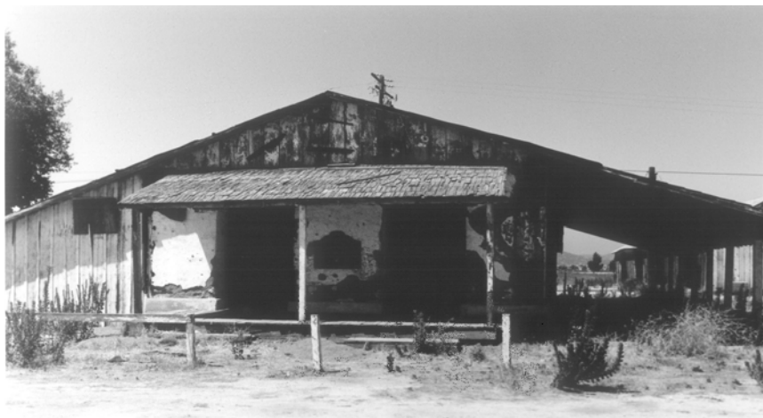
The Wolf Store before restoration work was done.
