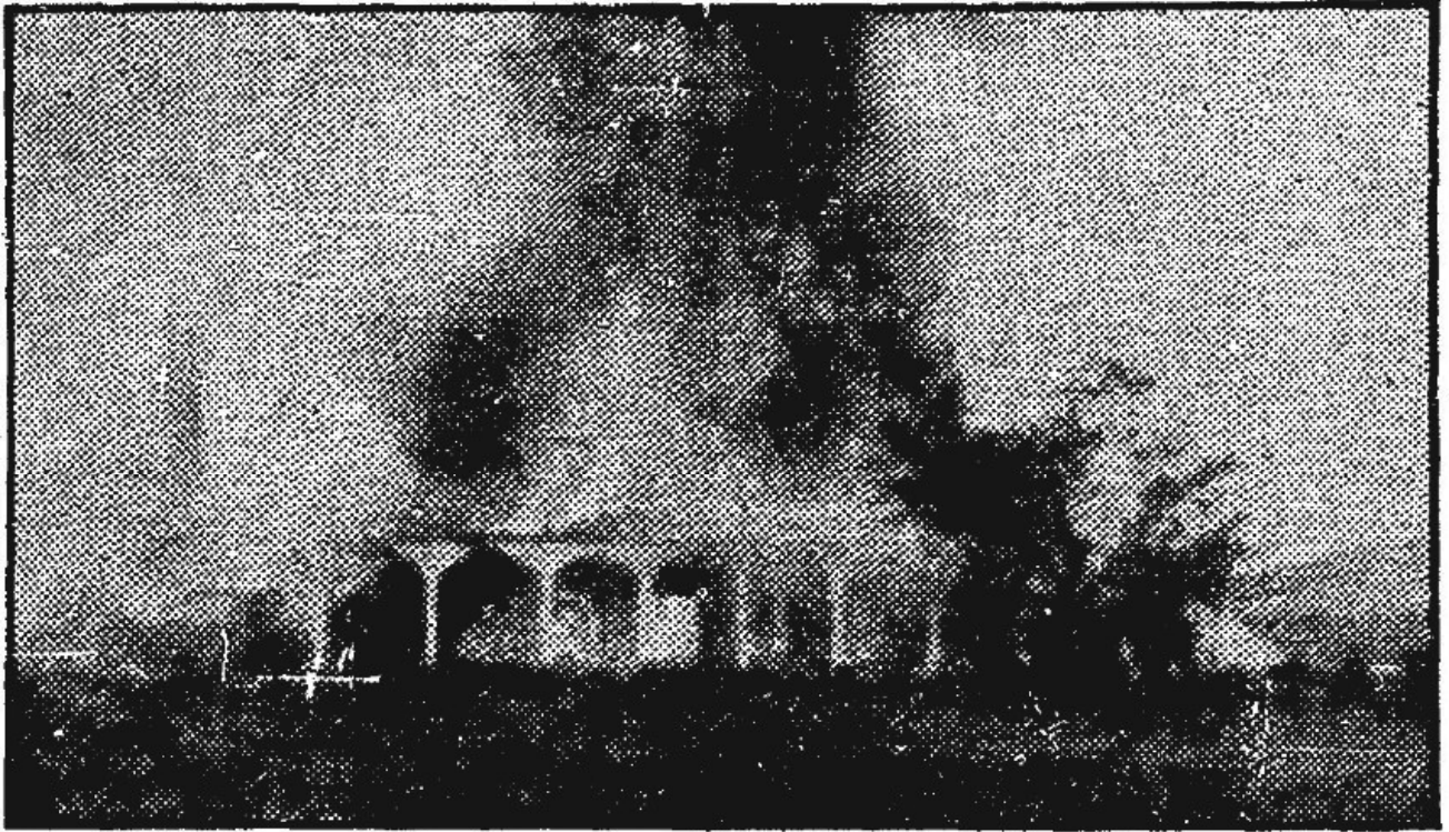
This fire at Stuhlman Hot Springs, near Murrieta, destroyed the main structure and threatened other nearby buildings. The blaze spread rapidly. Although handicapped by lack of water, volunteer firemen put up a valiant fight to save the structure, which was completed only last year.
