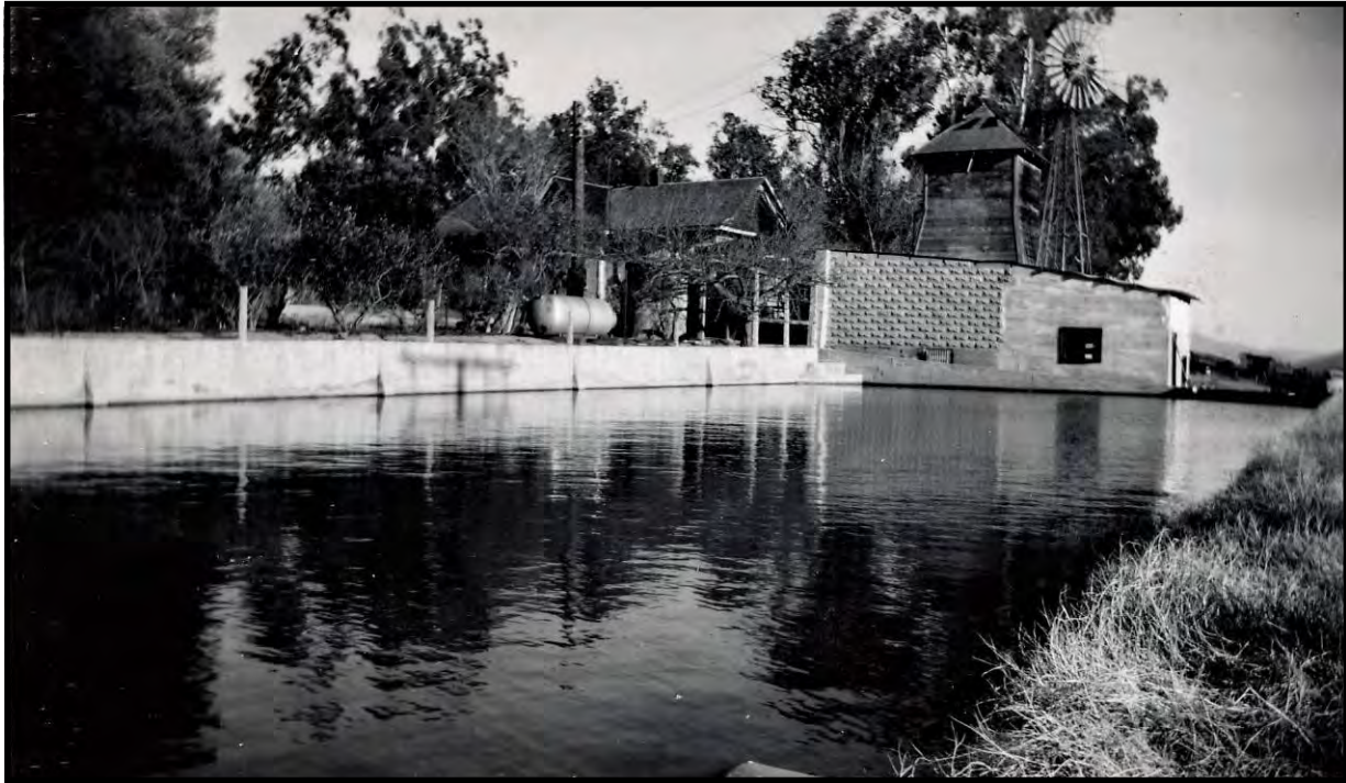
The Sykes Ranch reservoir, tank house, and farm house. The reservoir was built around 1924. It was 109 feet by 54 feet and 6 feet deep. Source: The Sykes Family Collection
