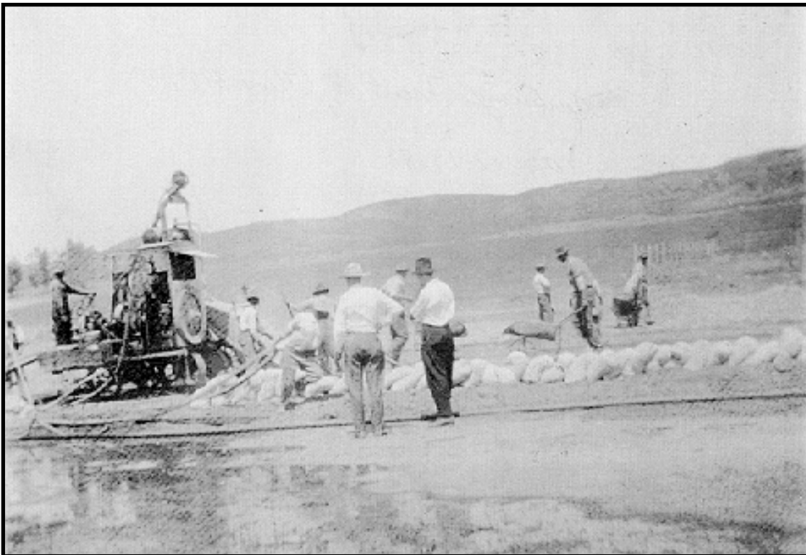
A road crew is laying cement on Front Street in Temecula in 1915 as a part of the Inland Highway construction project. (Source: The Gene Knott collection )
